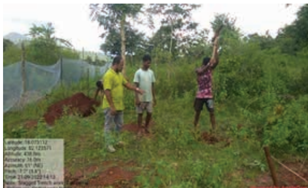
Staggered trench work at Pallam VSS, Malkangiri
