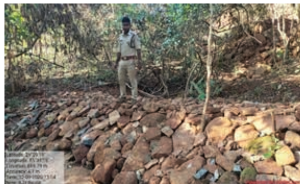
LBCD work at Raidiha VSS in Keonjhar Division
