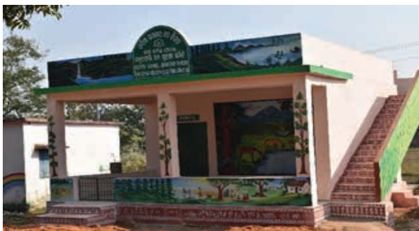
Thakurpali VSS Building, Deogarh Division
